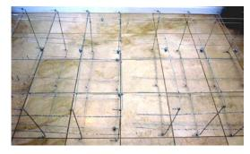
Be sure to feed the all of the legs of the extension cage **outside** the base cage. When clamping the Clips down, keep the overlap to a minimum as this directly affects the final cage height.
